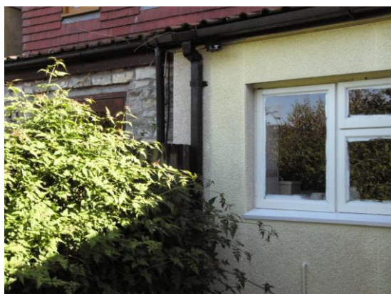
External insulation on the rear of the property
