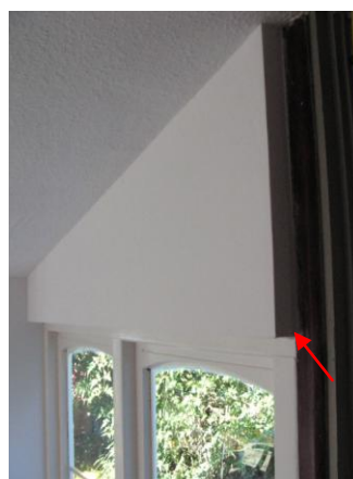
Internal wall insulation
