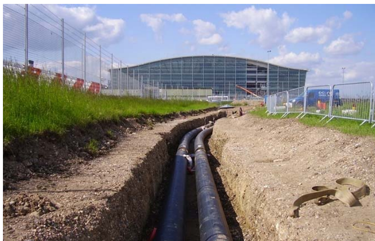
Figure 20: Heat main pipework at Heathrow Airport, Terminal 5 [© Vital Energi | www.vitalenergi.co.uk ]
