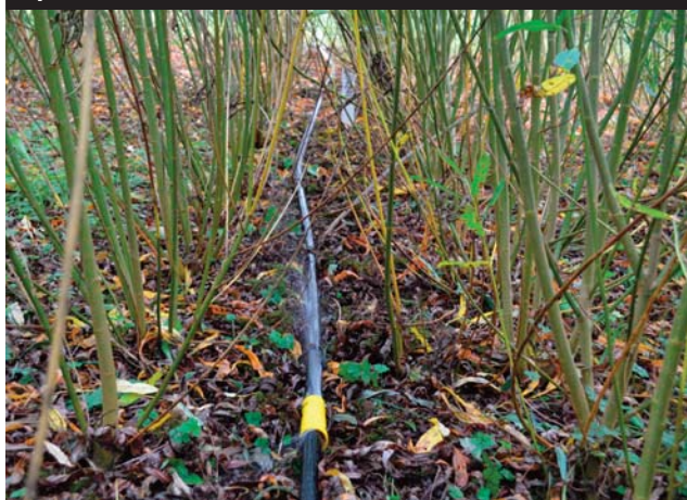
Pipework laid out within the double rows of willow
