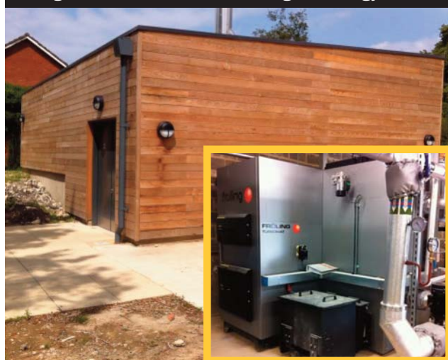
Froling Turbomat 320 kW boiler. Image: Econergy
