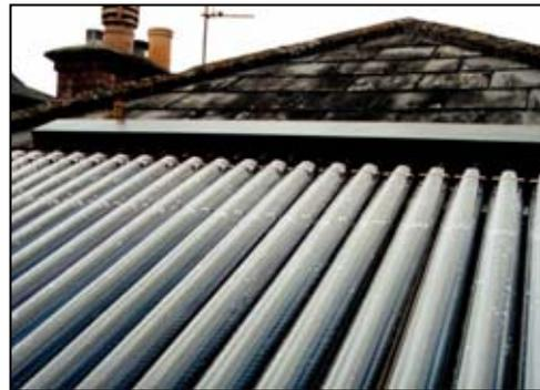
Figure 4.5: Evacuated tube collectors
