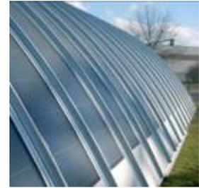
Figures 4.8 & 4.9 – ‘AluPlusSolar’ standing seam PV (amorphous)
