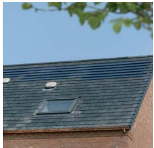
Figures 4.12 & 4.13 – C21 BIPV roof tiles (polycrystalline)
