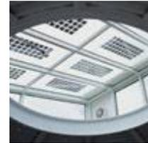
Figure 4.10 (left) & 4.11 (above) – translucent BIPV for rooflights/flat roofs
