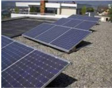
Figure 4.7 - console mounted panels on flat (monocrystalline)
