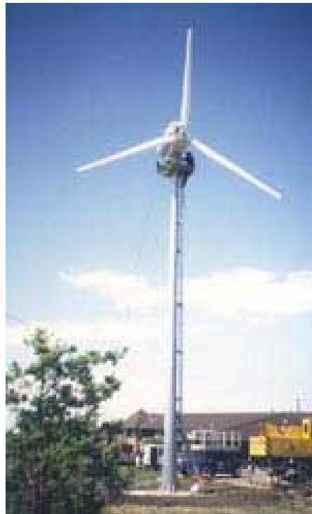
Fig D: Gazelle 20kW on 15m mast
