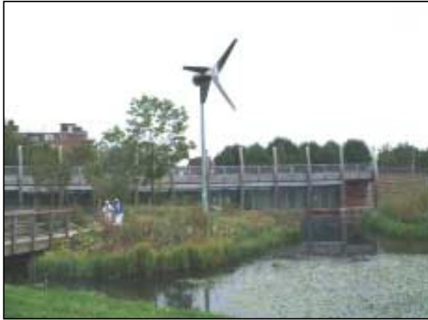
*Fig A: Proven WT6000 (6kW) on 15m mast*
