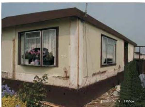
**Figure 1: Uninsulated single unit<sup>1</sup>**
