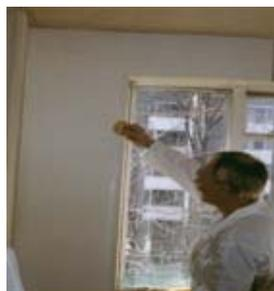
Use SEMPATAP EDGING TAPE to achieve a neat finish on all outward facing corners, window reveals, window heads etc. Cut SEMPATAP EDGING TAPE to required length, fold along the aluminium crease line to form a right angle with the aluminium facing inside. Brush SEMPATAP ADHESIVE along aluminium and the paper and leave to soak for a couple of minutes. Locate over the corner of the SEMPATAP THERMAL and smooth out. Remove excess adhesive with a damp cloth and leave to dry
