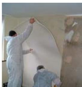
SEMPATAP THERMAL is applied foam side to the wall or ceiling. Cut SEMPATAP THERMAL to required length allowing 25mm overlap at each end then roll up with foam side facing out. Apply to wet adhesive on the top of the wall at the junction with the ceiling or to the ceiling at the junction with the wall then roll out and smooth with light level pressure.
