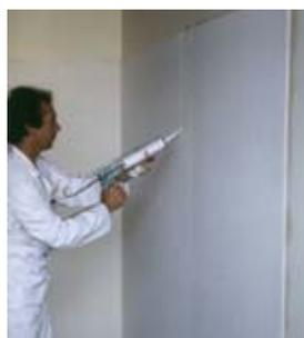
Gun the SEMPATAP SEALANT into all joints between the SEMPATAP THERMAL lengths where the adhesive has settled back during drying. Also, use to achieve a neat finish at the wall/ceiling junction and skirting. Wipe off any excess. When dry, if necessary, fill any sealant shrinkage with proprietary filler to totally hide joins.
