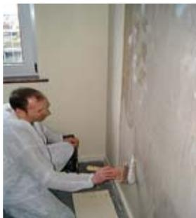
Remove any wallpaper and prepare the walls and ceilings as though you were going to decorate. Apply a liberal coat of SEMPATAP ADHESIVE to the wall or ceiling using the notched SEMPATAP ADHESIVE SPREADER. Only apply the adhesive to one drop length area at a time.
