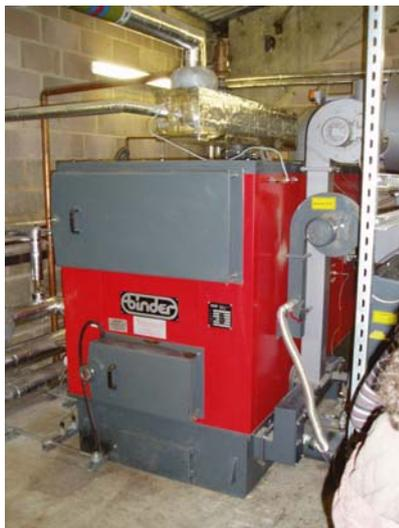
***Figure 4: 150kW wood chip boiler heating a leisure complex***
