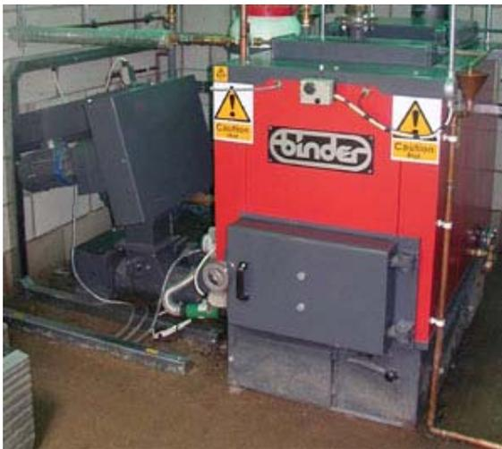
**Figure 8: Binder (50kW) wood chip boiler meets 50% of large educational centre's heating requirement**
