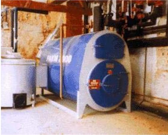
**Figure 6: Farm 2000 boiler suitable for heating farm buildings and estates; will burn a variety of fuels**
