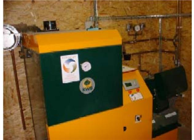
**Figure 7: KWB (25kW) woodchip boiler heating an organic farm shop**
