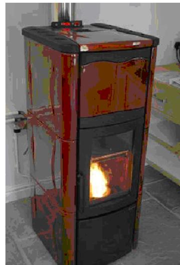
***Figure 5: A small (22kW) stove with back up boiler heating a farm house***
