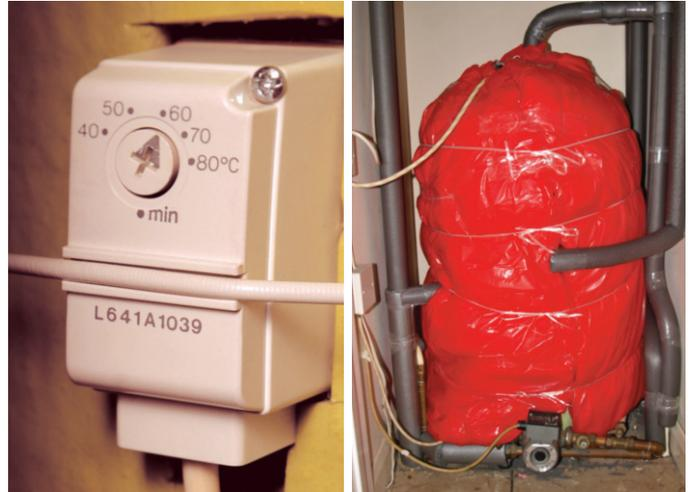
A cylinder thermostat (left) will stop you wasting money on overheating your water, while to save more on water heating, make sure you get your hot water cylinder and pipes insulated too
