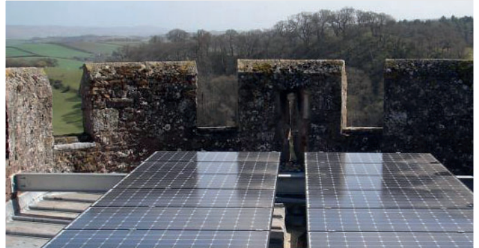
The National Trust continues to exploring all sorts of ways to generate energy at its properties, from solar (pictured) to hydro and biomass to air source heat pumps.
