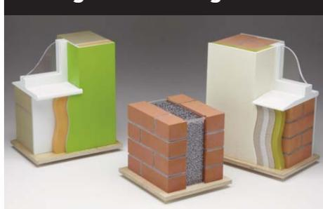
We designed these 1:2 scale models of wall insulation types for our own outreach, but they've proven so popular that we've since sold sets to a dozen community groups for engaging with the public around local energy efficiency programmes. From L to R: solid wall insulation (internal); cavity wall insulation; solid wall insulation (external).
