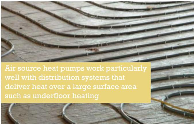
Air source heat pumps work particularly well with distribution systems that deliver heat over a large surface area such as underfloor heating
