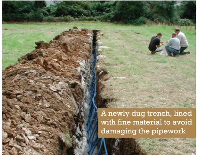
A newly dug trench, lined with fine material to avoid damaging the pipework
