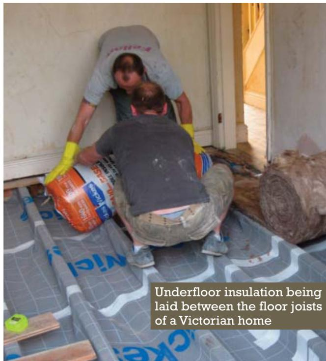
Underfloor insulation being laid between the floor joists of a Victorian home
