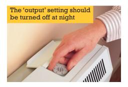
The **boost** setting can be used to throw out extra warmth. But it uses expensive peak rate electricity. Use all the stored heat first by opening the output fully before using boost.
