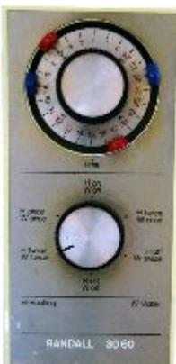
Try setting the timer for an hour in the morning and an hour in the evening. If you don't run out of hot water, that will be enough.
