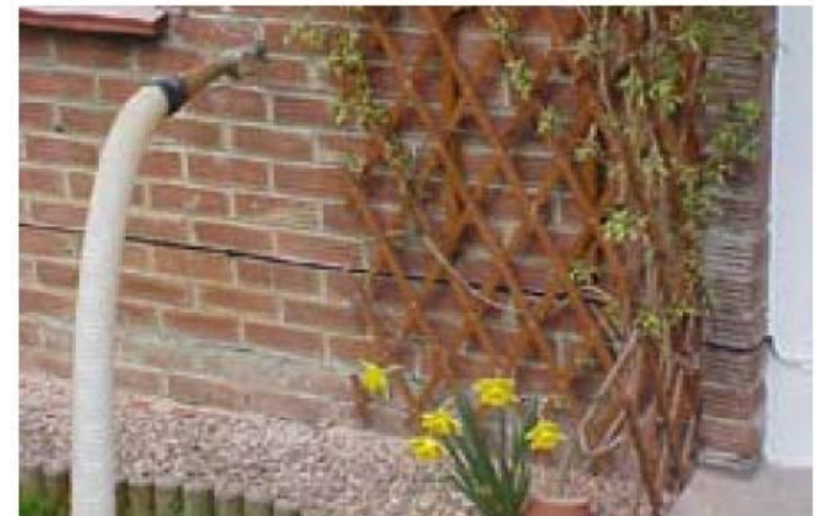
Insulation being injected into the wall
