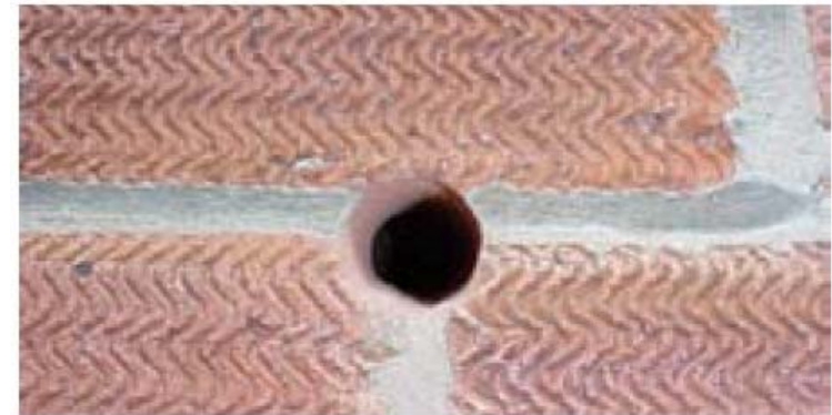
An injection hole prior to filling
