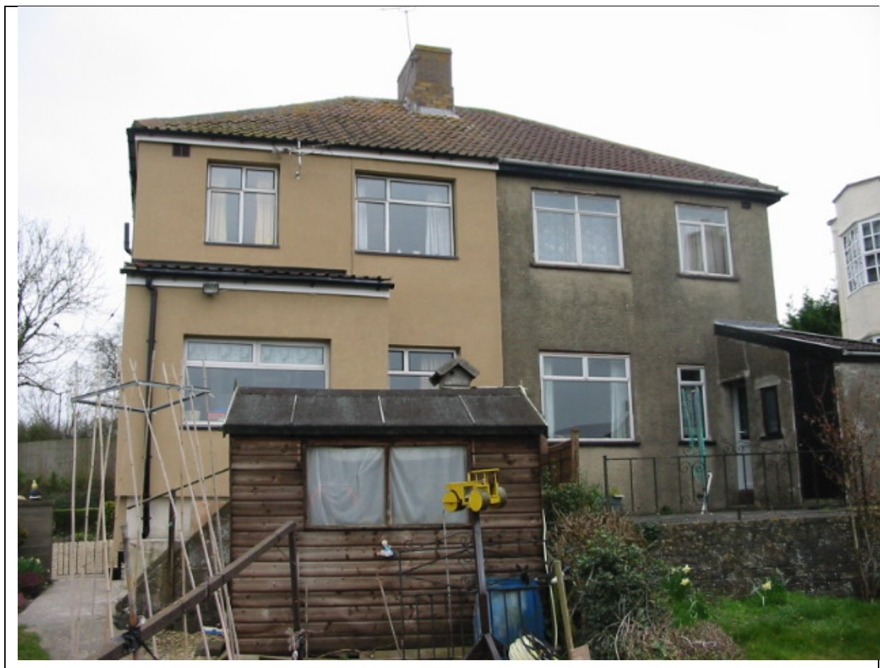
Figure 13: SWI improves the appearance of the home as demonstrated by C20's completed installation in comparison with the other half of the semi-detached dwelling.
