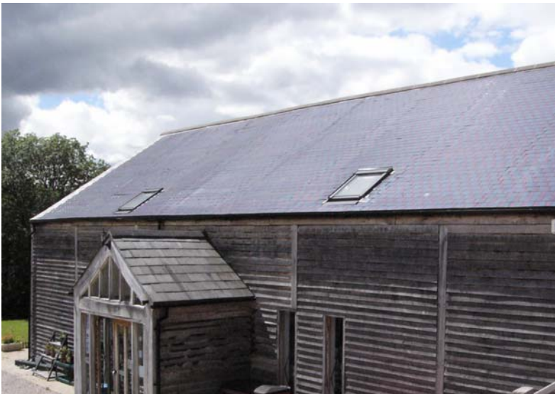
Figure 5.21 When are heritage solar tiles acceptable on visible roofs of traditional buildings in Bath? (workshop participants)
