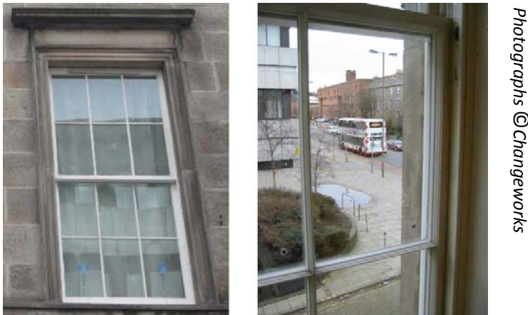
Figure 5.4 When is slimline double glazing acceptable for traditional buildings in Bath? (workshop participants)
