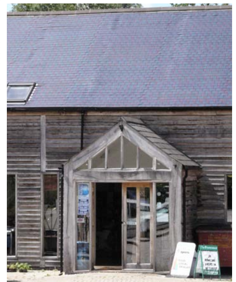
Community shops like this one, with its roof of solar tiles, is the kind of initiative that the Levels and Moors energy project seeks to promote
