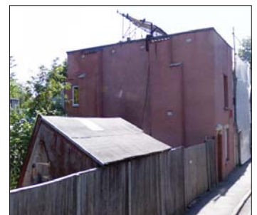
The original building in Philip Street in it's hey-day, and (below) the house as it looks today
