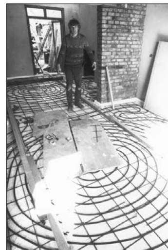
Underfloor heating being installed at the Philip Street premises
